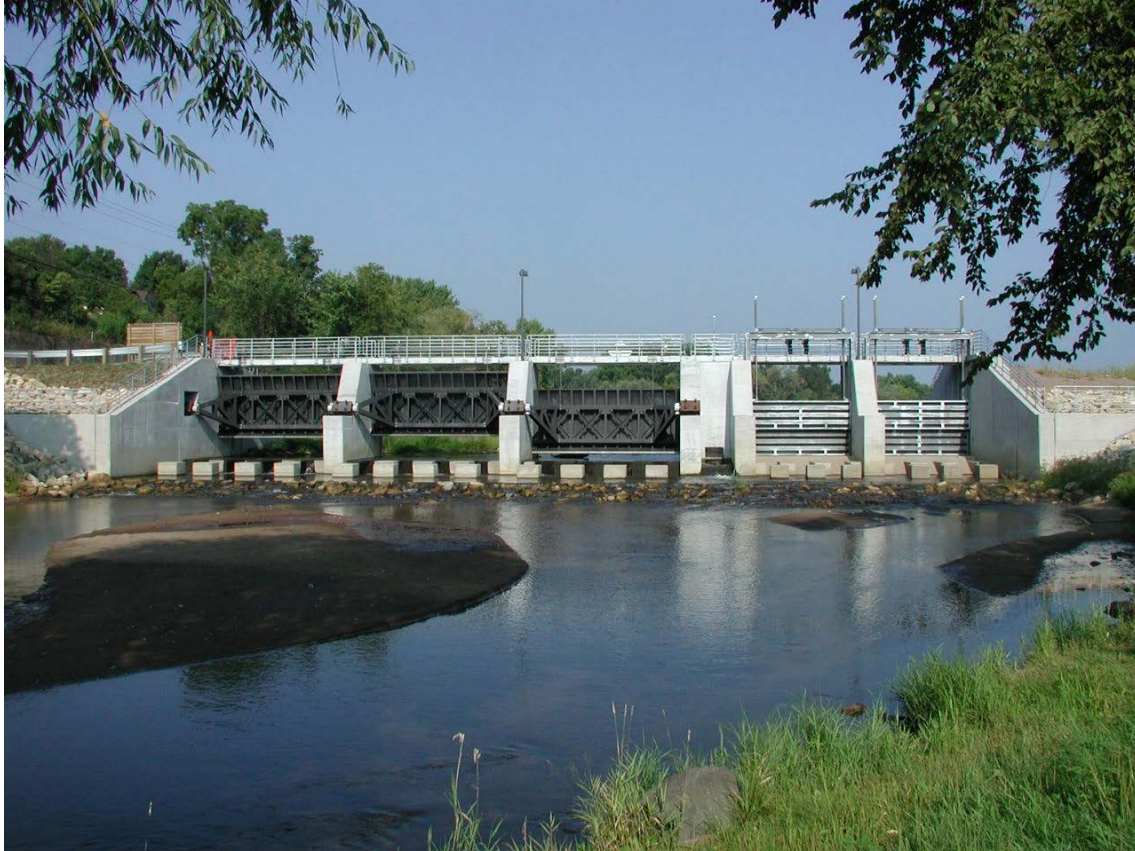
Figure 4: Two installed split-leaf gates (right side of photo) in Bloomer, WI (Photo: Ayres)
