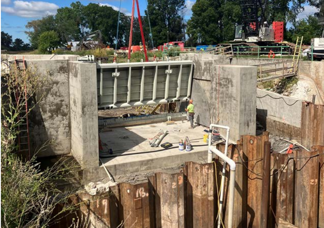
Figure 2. Crest gate being installed in new spillway at Sheboygan Marsh (Photo: Aaron Brault)
