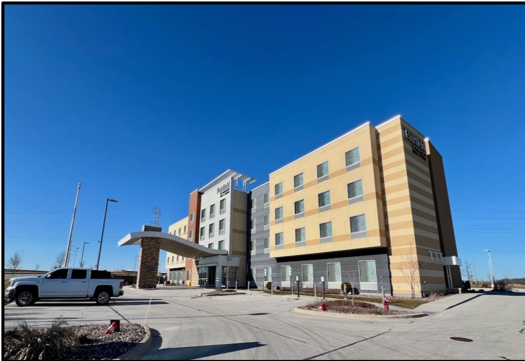
Fairfield Inn & Suites – 4117 S. Taylor Drive, Sheboygan
